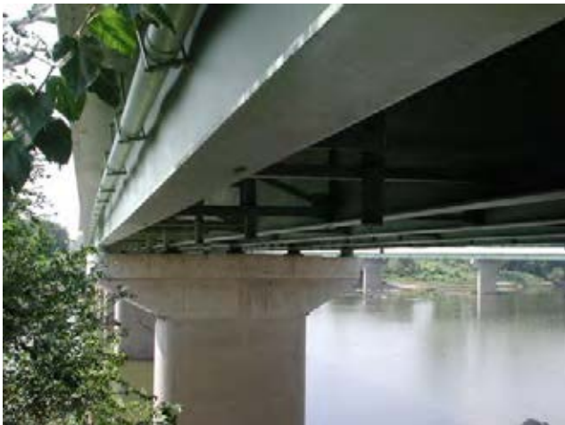
View of the underside of the eastbound U. S. 40/ National Road bridge. Source: Storrow Kinsella Associates Inc
