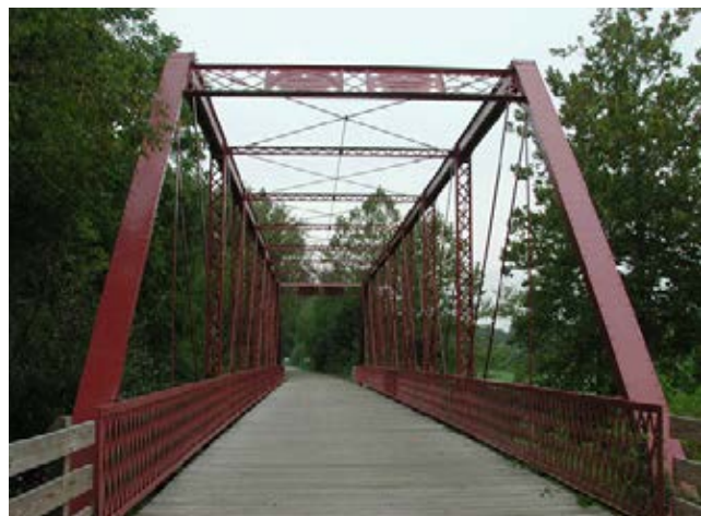
Relocated bridge, now used for the Clear Creek Trail in Bloomington, Indiana. Photo courtesy of Storrow Kinsella Associates Inc.
