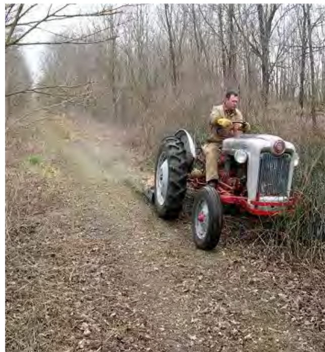
Volunteers help clear the corridor, preparing it for use. Photo courtesy of National Road Heritage Trail, Inc.
