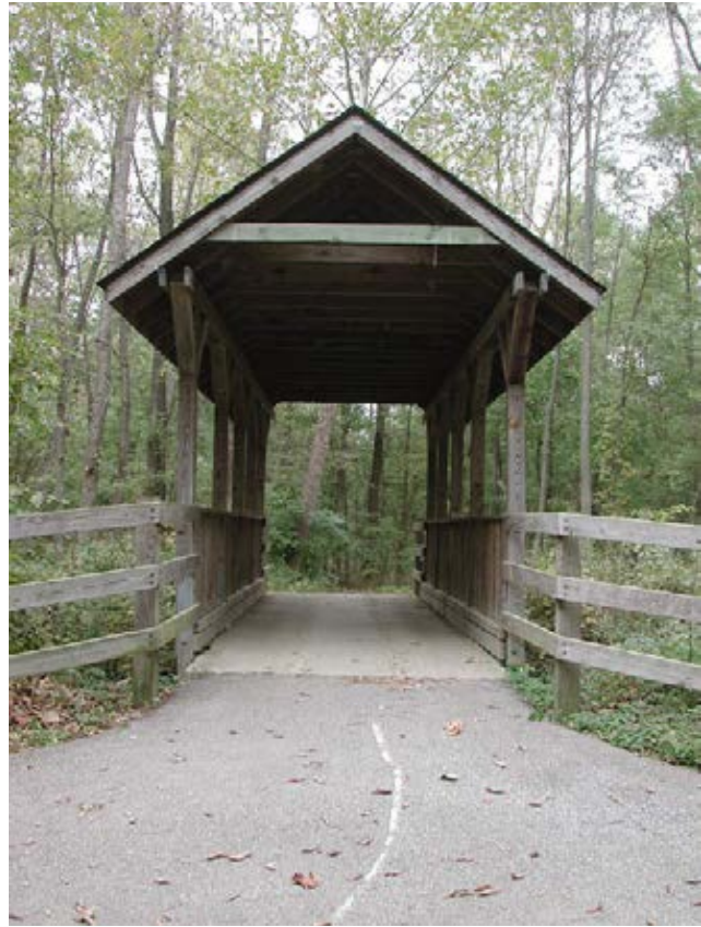
This is an example of a newly constructed bridge for a trail crossing a stream. Photo courtesy of Storrow Kinsella Associates Inc.
