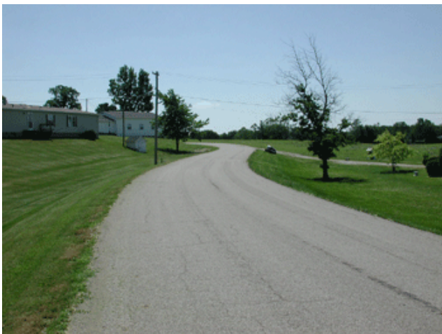
Historic National Road in Dublin. Source: Storrow Kinsella Associates Inc
