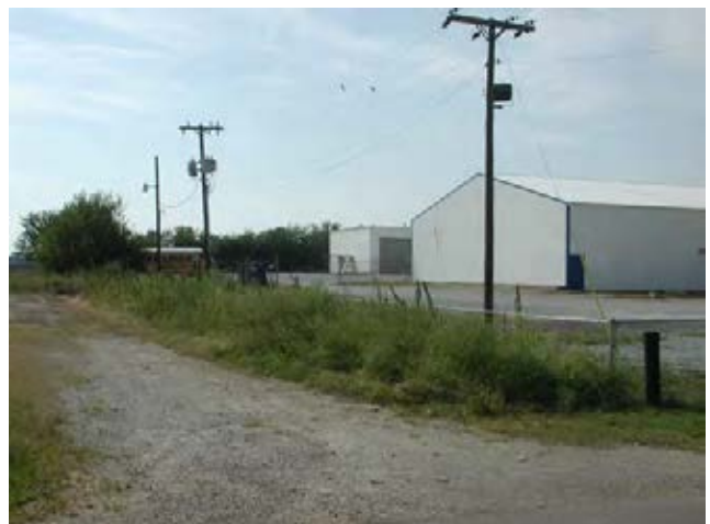
View from C. R. 400 E looking west. Source: Storrow Kinsella Associates Inc
