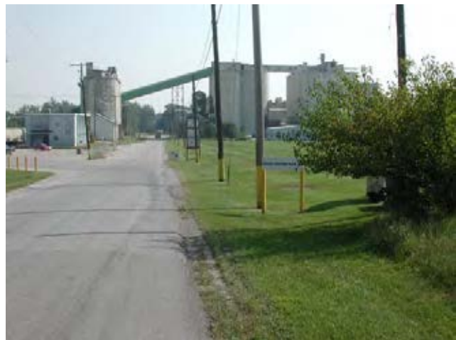
View looking south along C. R. 150 W, at the approximate location of the proposed trail crossing. Source: Storrow Kinsella Associates Inc
