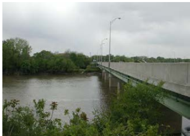
The U. S. 40/National Road bridge spans the Wabash River west of Terre Haute. Source: Storrow Kinsella Associates Inc
